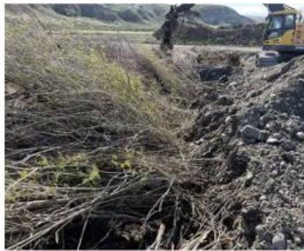
STAGE 2: VERTICAL SLASH/RACKING PLACED AND BACKFILLING TRENCH WITH NATIVE ALLUVIUM.
