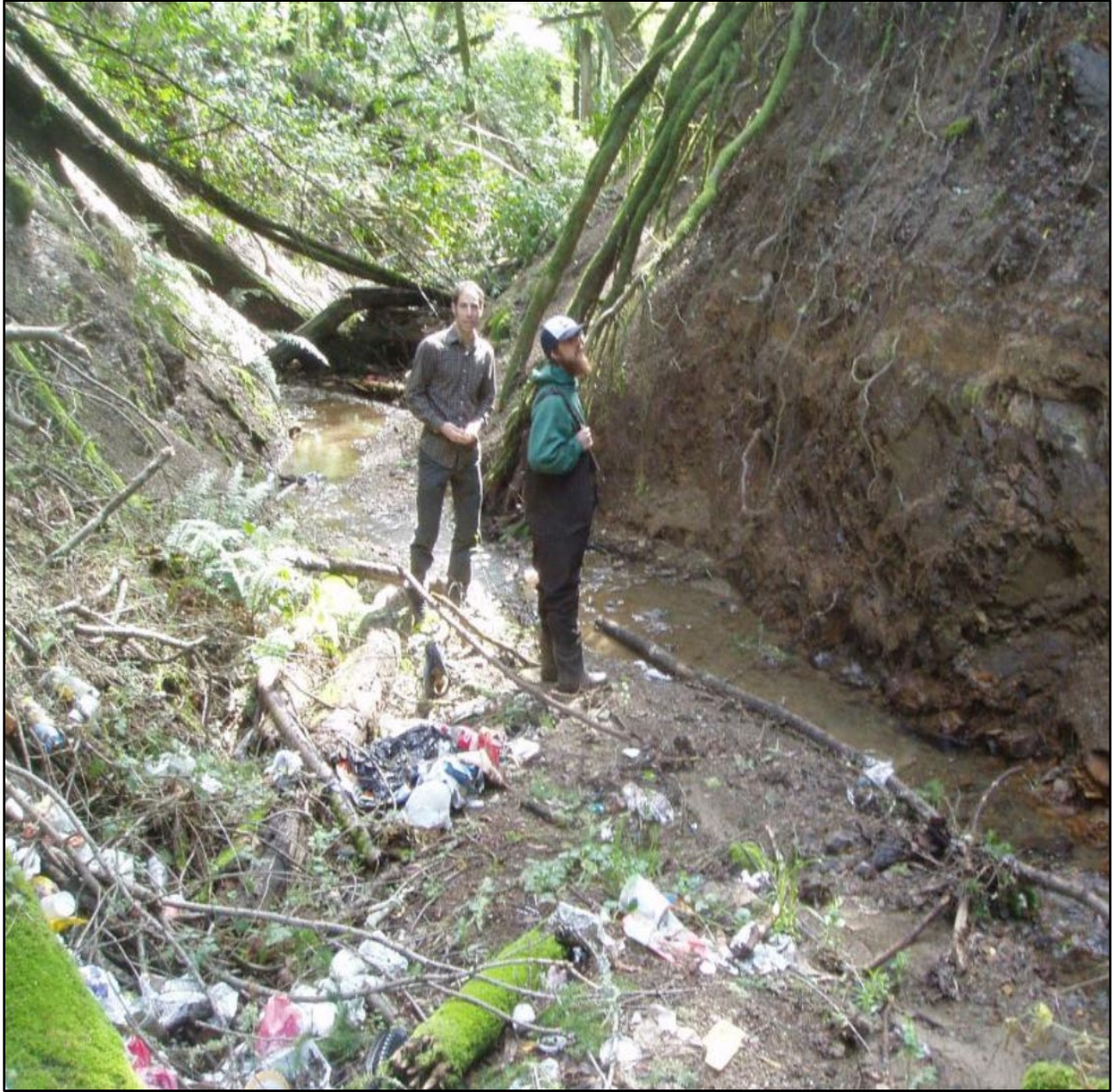
Figure 11. Deep incision and trash dump, Purrington Creek at Graton Road pullout (OEI SHaRP presentation 2022).
