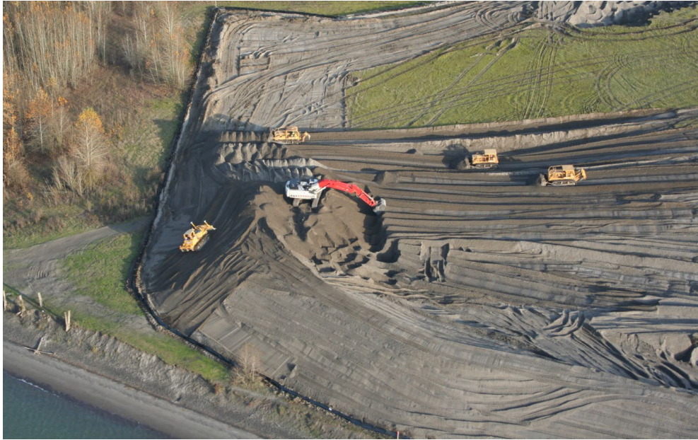
Figure 1-6. Outer berm construction at an upland placement site.
