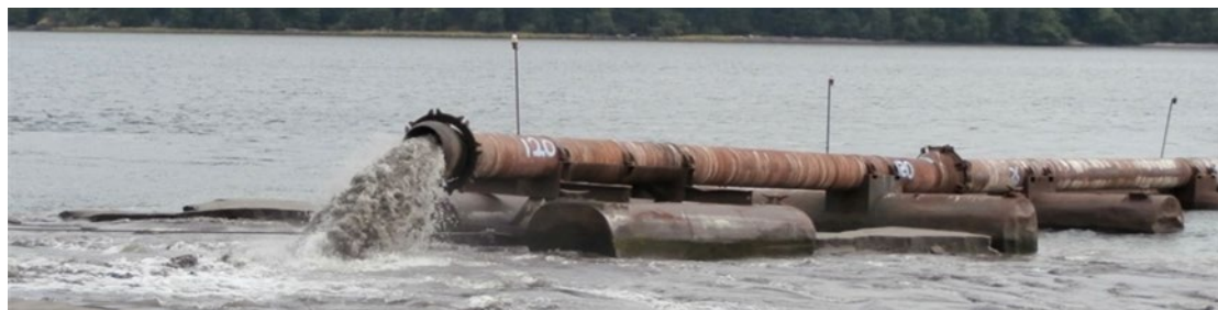
Figure 1-10. Shallow water placement operations.
