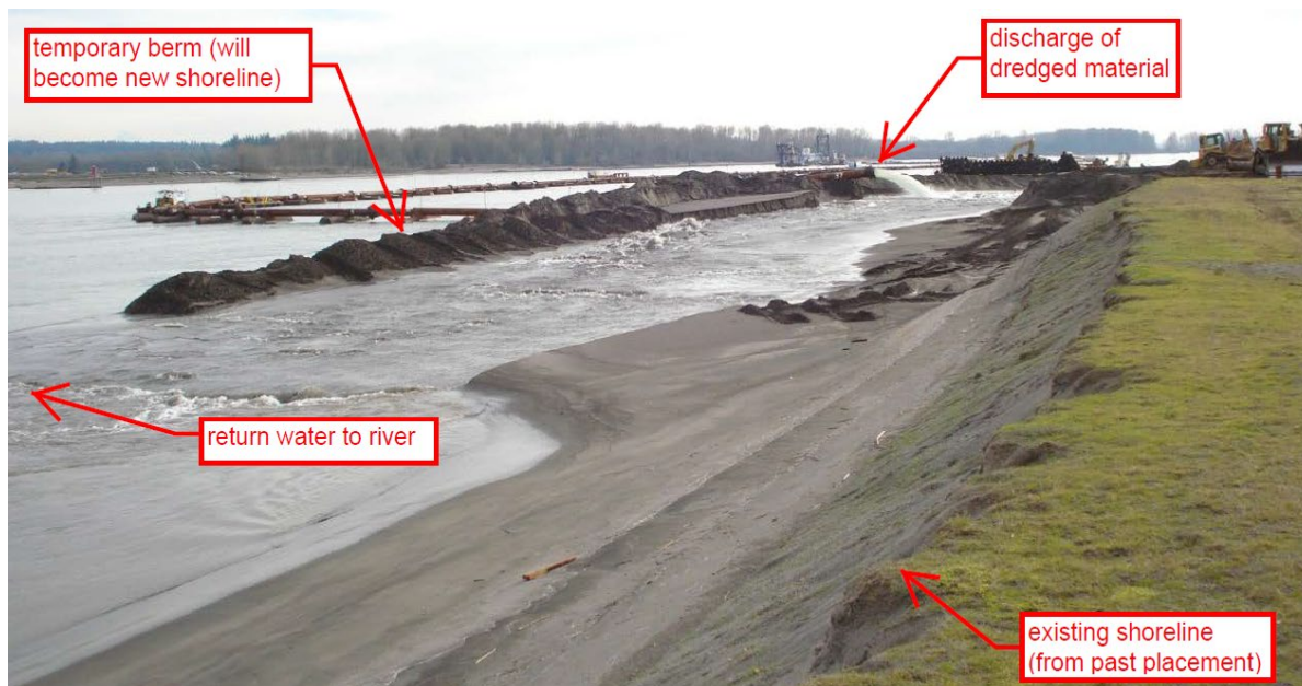
Figure 1-9. Overview of typical shoreline placement with interim berm created from dredged material.
