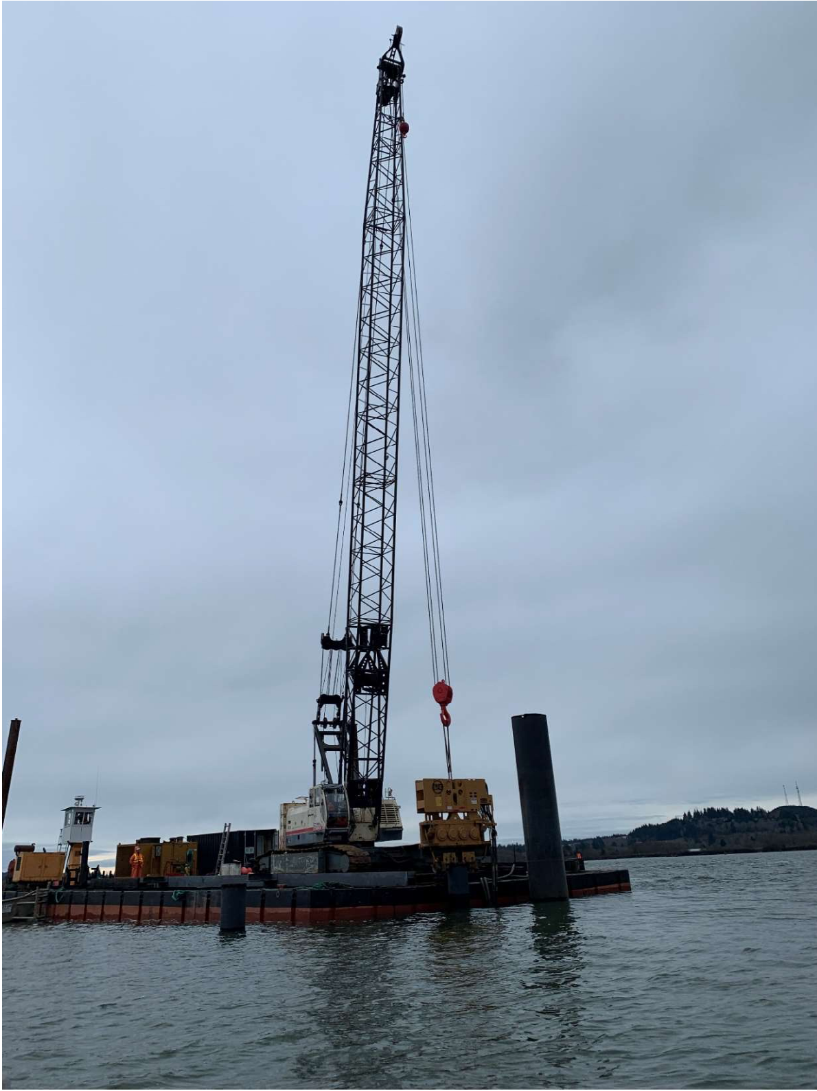
Figure 4. Vibratory Hammer Removal Operation on 24-Inch Piling
