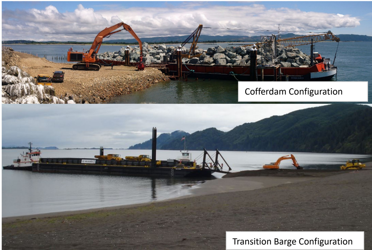
Figure 7. Example Photos of Typical Barge Landings.
