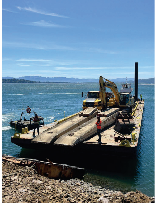
Enclosure 1. Ballard barge for offloading material at the Tillamook South Jetty project.
