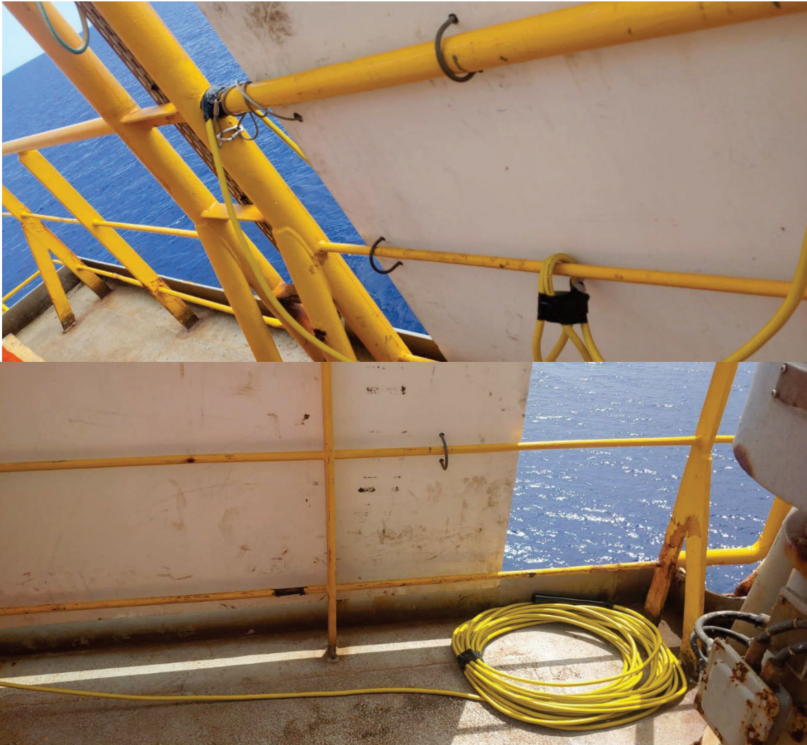
Figure 1: PAM cable deployment
