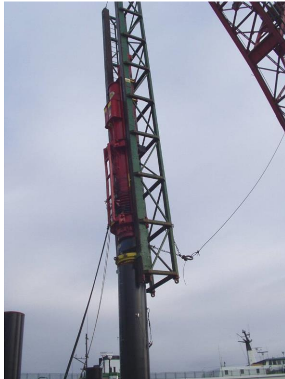
Figure 1-5 Impact Hammer Driving a Steel Pile
