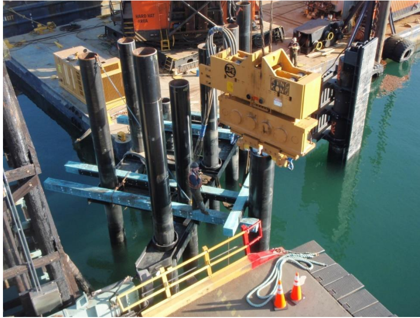
Figure 1-4 Vibratory Hammer Driving a Steel Pile
